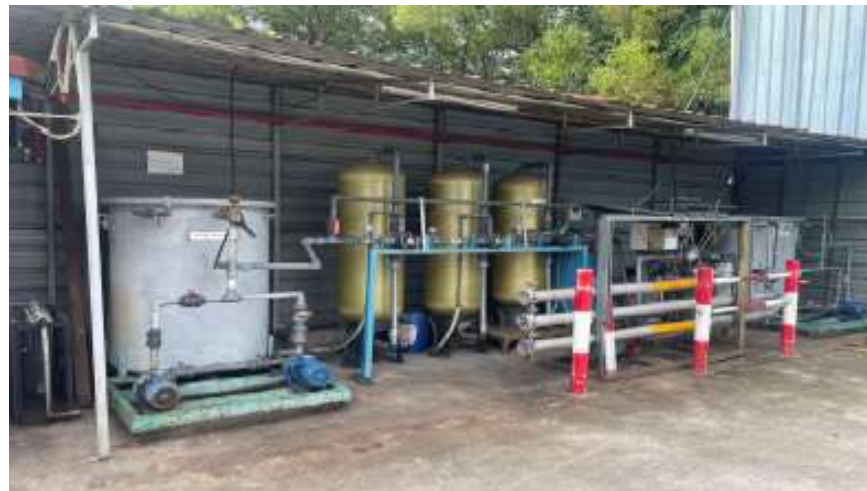
In-house RO Plant to support DI Washing Line
